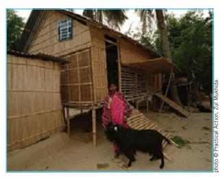
This house on a char (river sandbank) near Faridpur, Bangladesh is built on posts to cope with flooding
